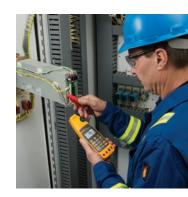
Measure process and other automation 4 to 20 mA signals without breaking the loop.
