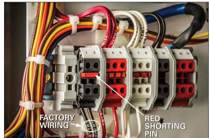
Figure 8. Terminal block TB1
