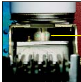
Contact Erosion Indicator
