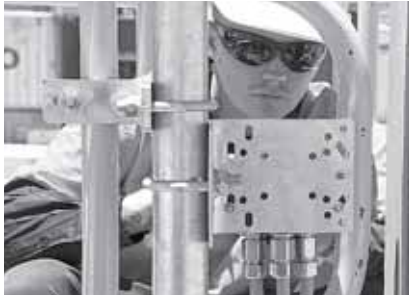
Optional raised junction box plate for easy termination and inspection
