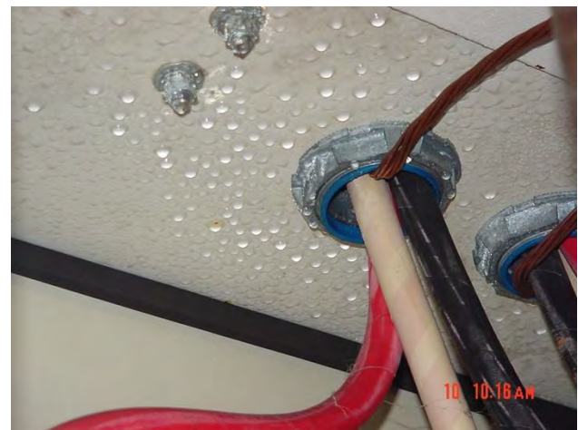
Figure 7. Condition that caused the unacceptable IRP
